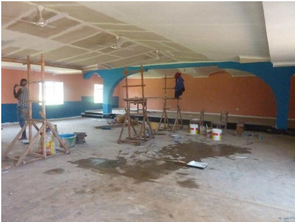
Figure 18 - Working on the new building for Salama Africa
