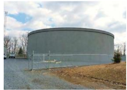
Figure 5: D-115 concrete premix tank (Rettew, n.d.)
