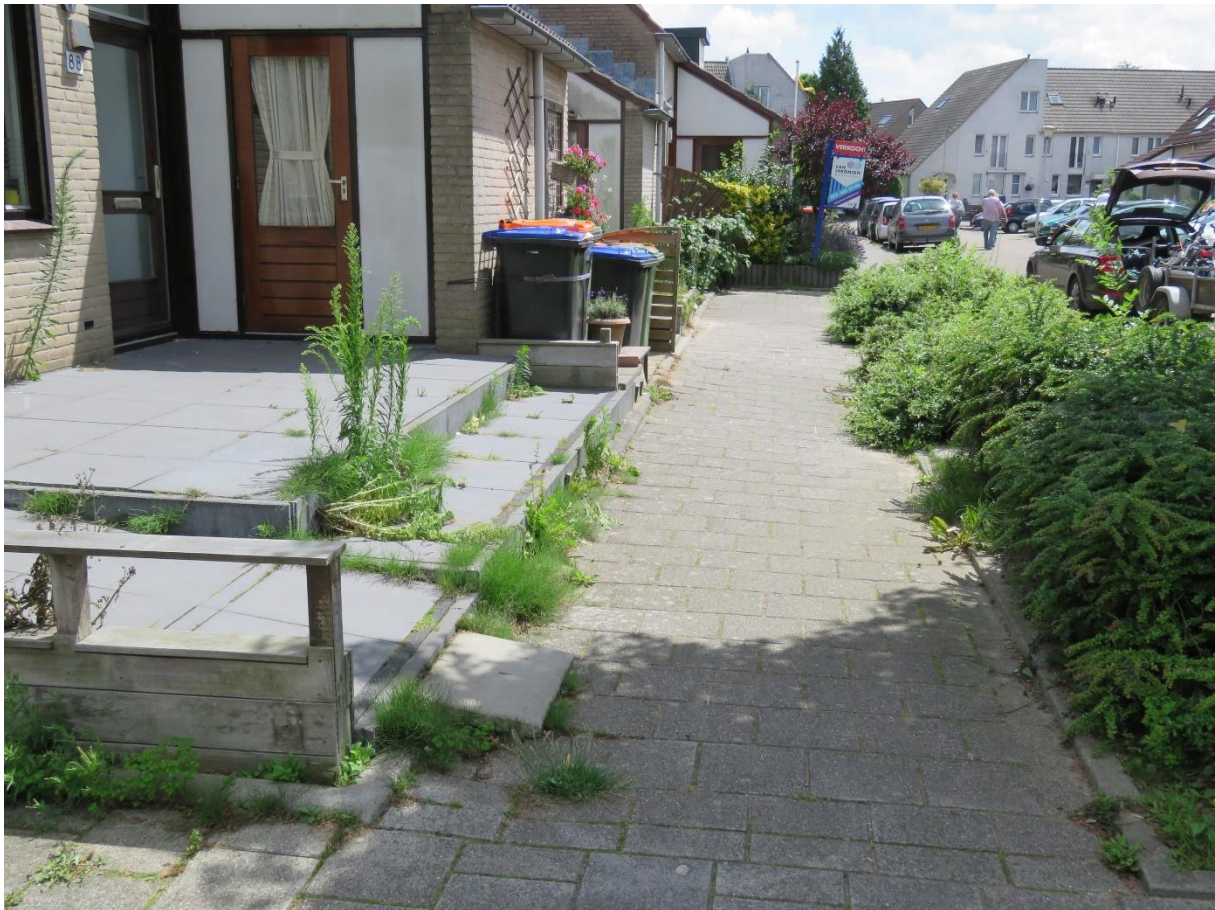
Image 9: The height difference between a reinforced house and a sidewalk. Due to this difference, the sewerage is damaged severely if no action is taken. (Gemeente Zwijndrecht, 2019).
