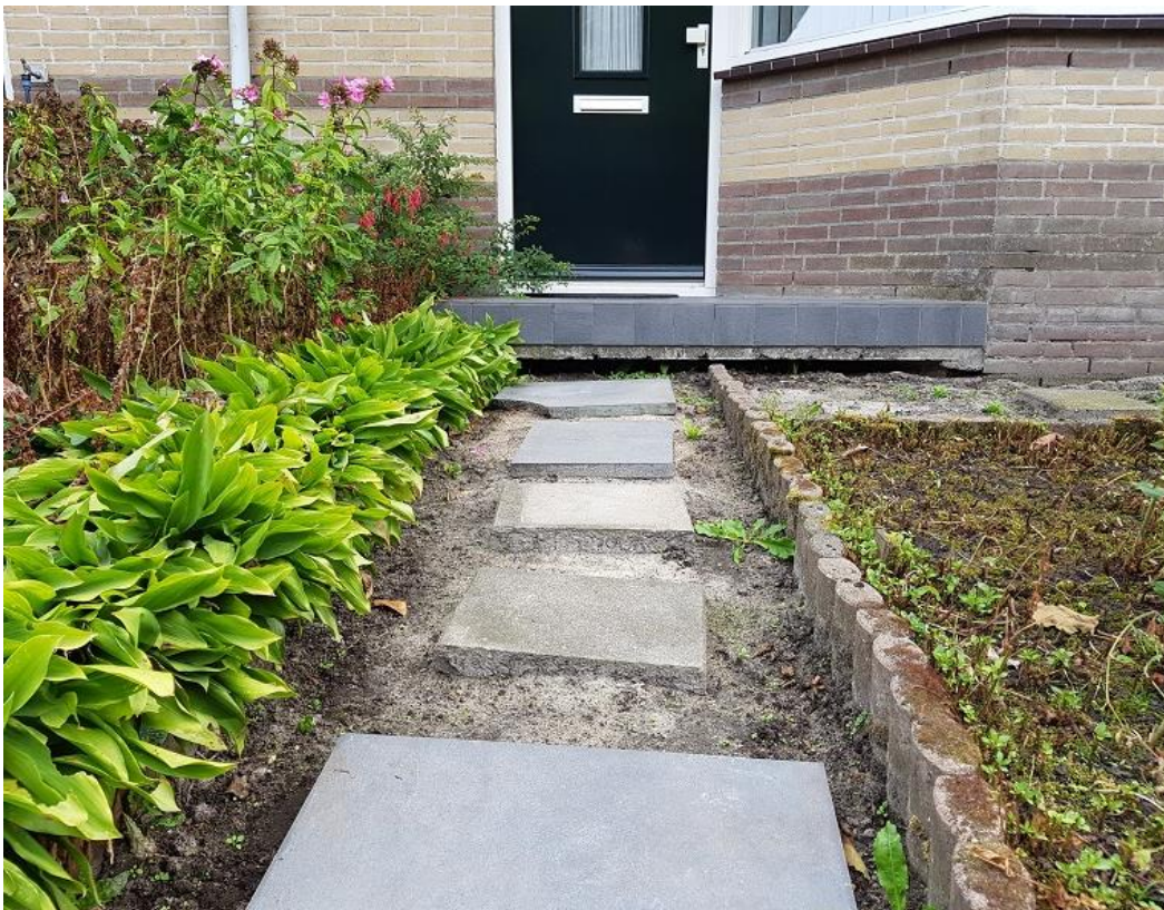
Image 10: The gardens are sagging while the houses remain at the same level. Source: Jos Scholman, 2019
