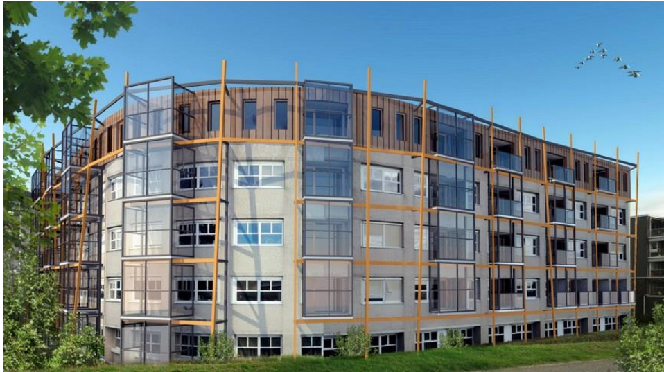
The Bakenmonde (A3 Architecten 2019)
