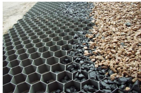
Figure 21 Permeable pavement used in example garden. Source: Lekker in je tuin (n.d.-b)
