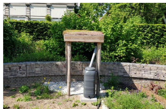
Figure 22 Construction connecting small green roof to rain barrel. Source: Lekker in je tuin (n.d.-b)
