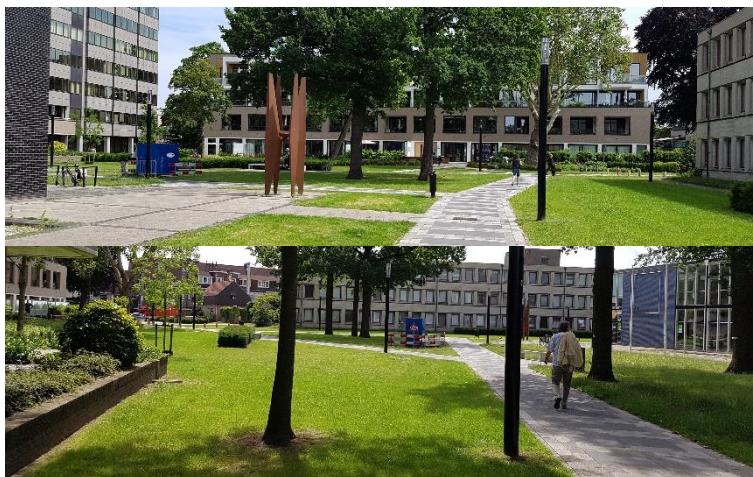
Figure 17 Impression of 'Zonnehof' square after urban renewal in 2019 (Source: Author, picture taken on 18/06/19)
