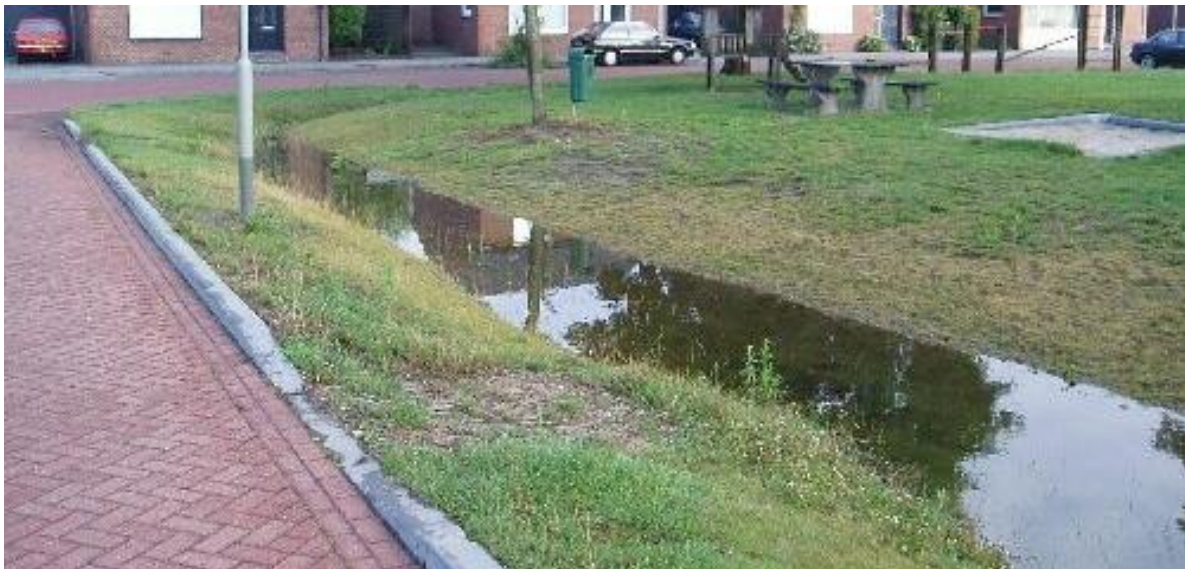
Figure 1 Example of a wadi in a residential area
