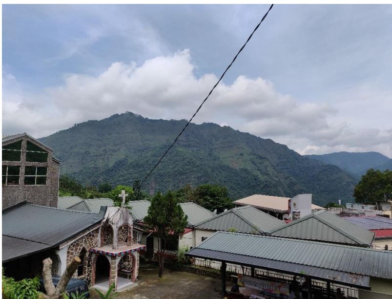
Figure 14: Xinmei Village, church on the left and part of the residential area on the right. Source: Author's research
