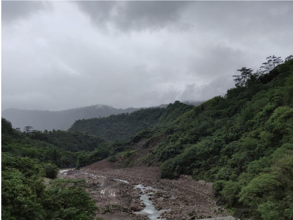
Figure 26: Before river clean-up, source: Author's research.
