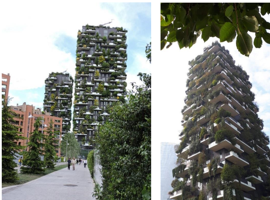
Figure 1: Left: The two towers of the Bosco Verticale in Milan, right: the façade of the Bosco Verticale
