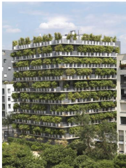
Figure 2: The Flower Tower in Paris, designed by Édouard François and arguably a predecessor of the vertical forest. Source: Maison Édouard François.
