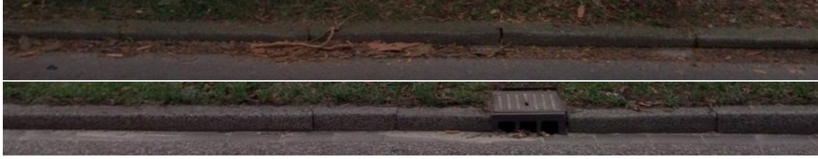
Figure 51: Two images of the sides of roads. Often, there is a significant amount of natural waste, or the paving is of a different material, like stone or brick . Water could also accumulate there, though CycloMedia usually drives in good weather. The fact that these road edges can deviate from the usual appearance of a road, it is likely that the network has most trouble with segmenting such edges.
