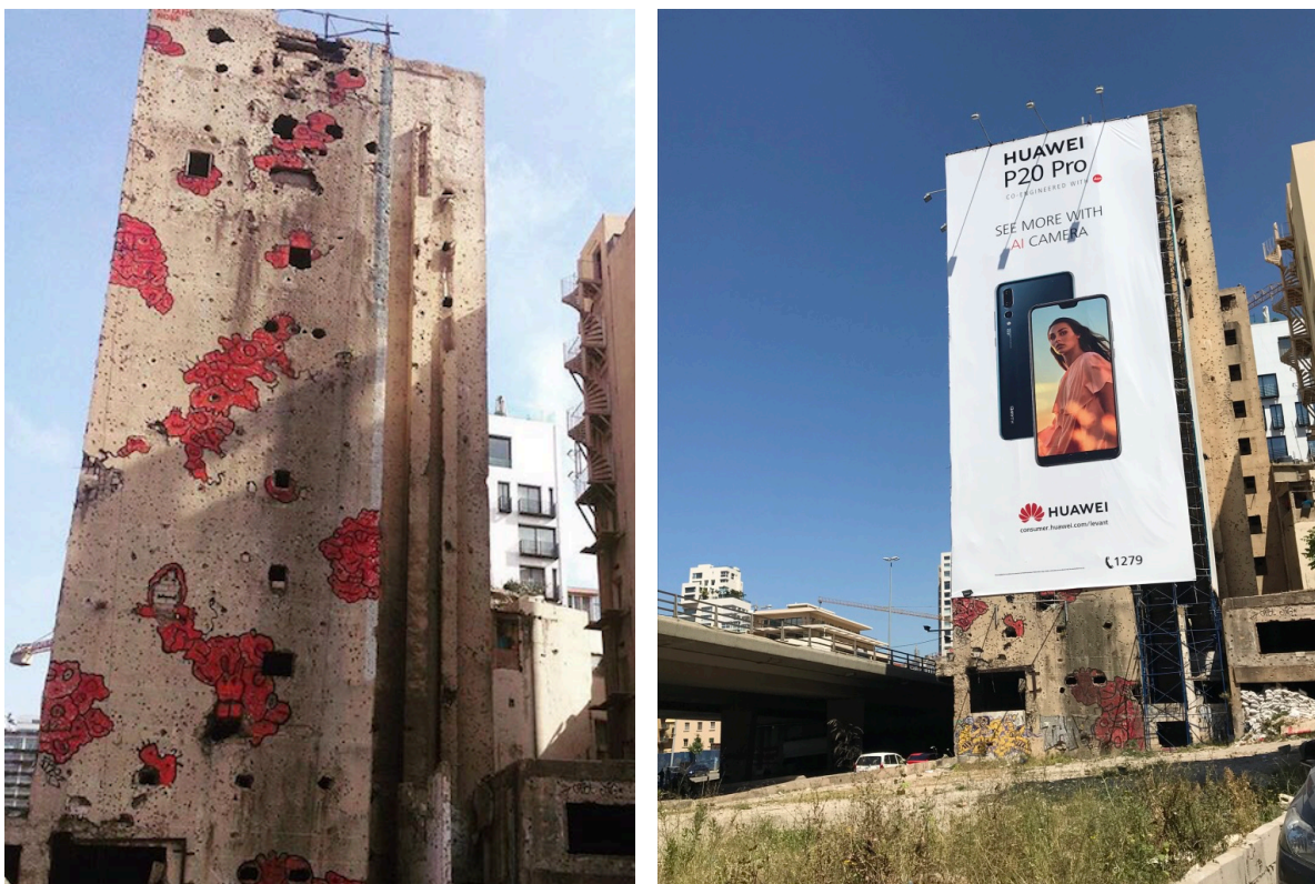
Image 1.1. Building next to the Fouad Chehab bridge
