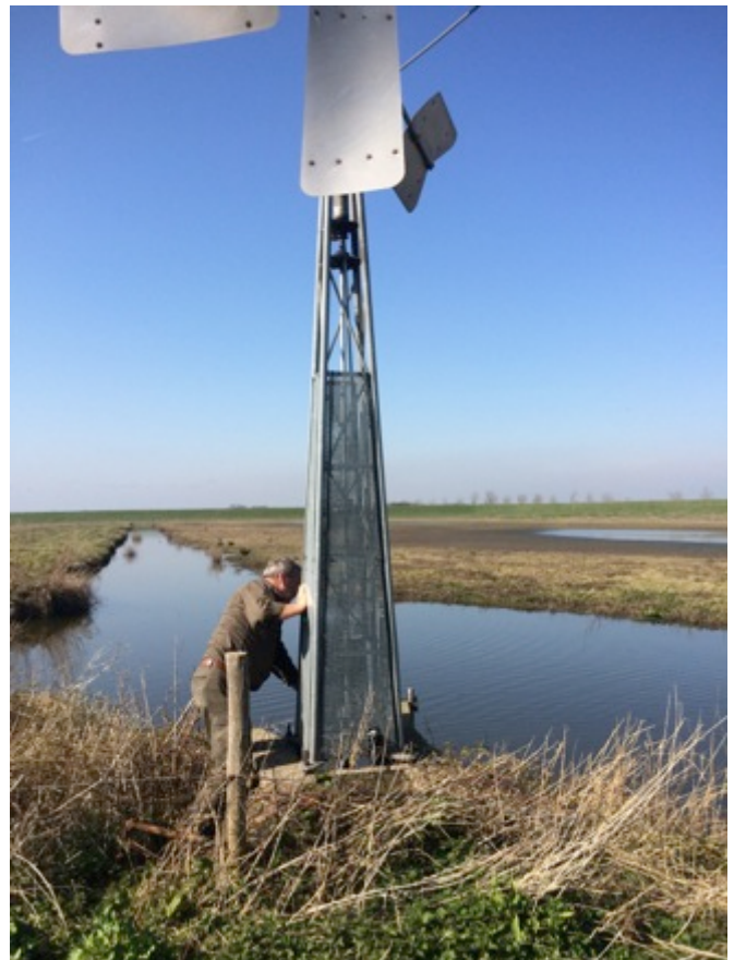
Ranger Eduard checking on the Bosmannetje - waterpump windmill or Tiengemeten in the weemoed area. The waterlevel was quite high therefore he suspected it defect. Picture taken by author.
