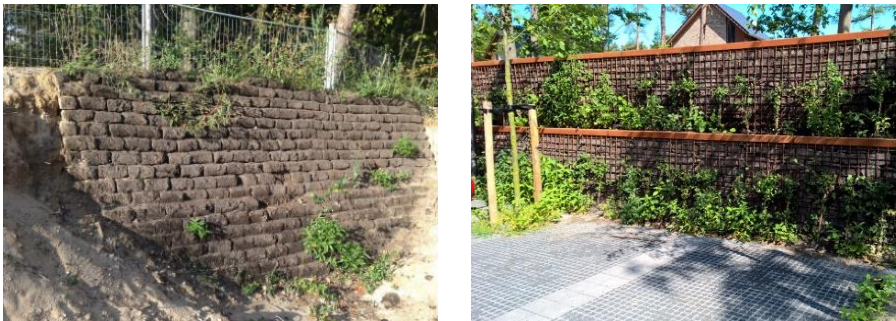
Figure 12. Learning-by-doing in case 3: adjustment of retaining structure intervention
