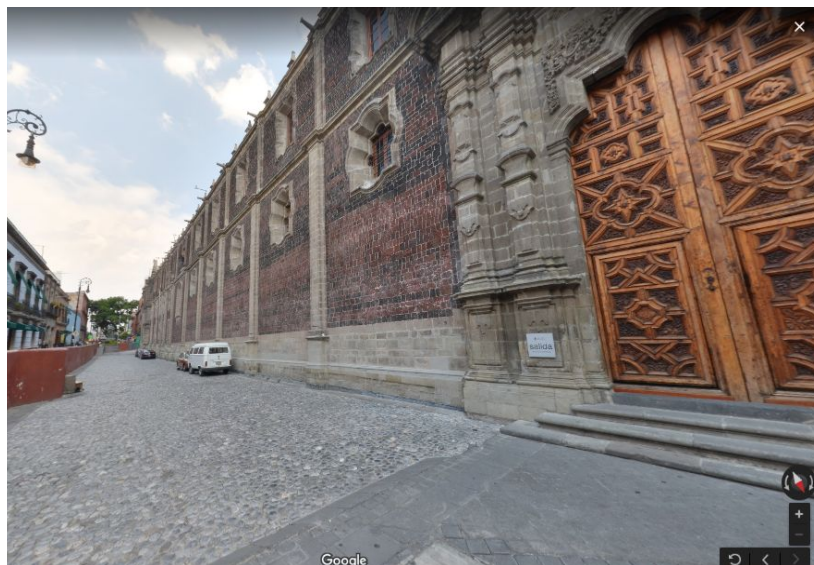
Figure 6.9. Facade of San Ildefonso College on San Ildefonso street, an example of a historic building with a closed facade with no points of refuge.
