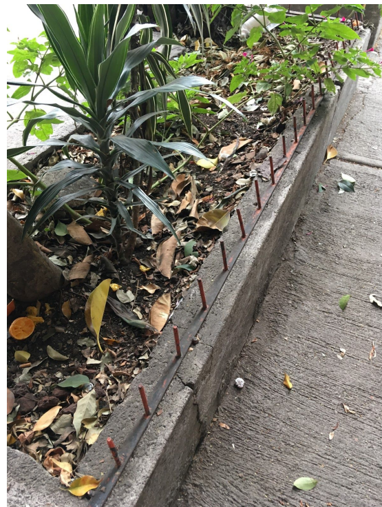
Figure 4.10. Urban equipment preventing residents from sitting on the curb: a hostile environment to women with children, wheelchairs, bags
