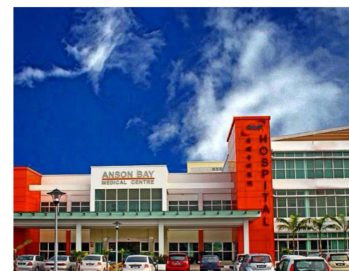
FIGURE 6 - ANSON BAY MEDICAL CENTRE (IMAGE FROM: HTTPS://WWW.FLICKR.COM/PHOTOS/ZAIMHQ/15724872093 )
