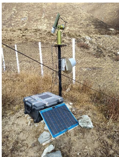
Figure 11: AERONET station at Kyanjin
