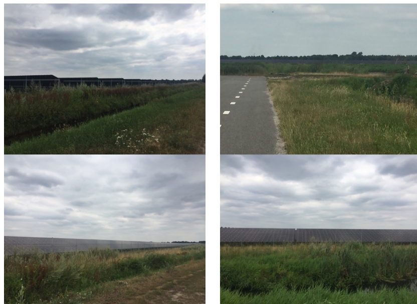
Fig 6. The views of solar park Lange Runde with different angles and distances
