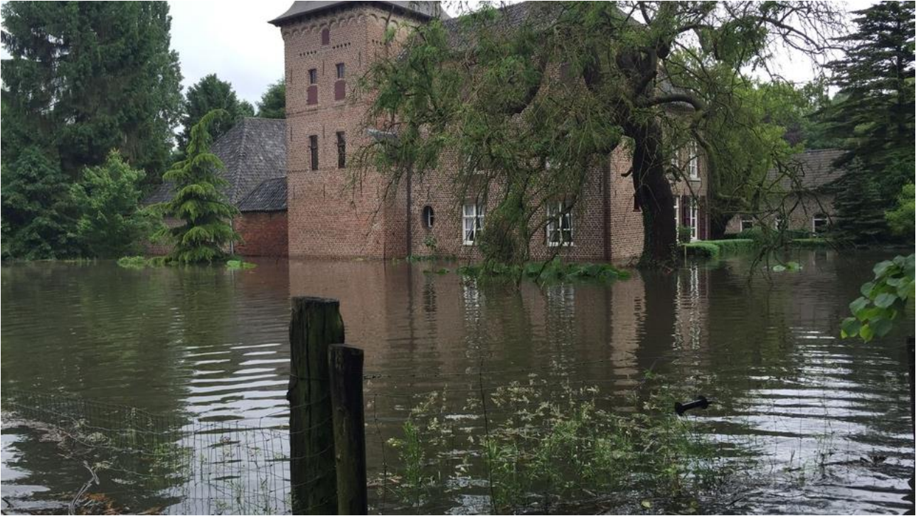
Figure 3 - Tegelarije Castle Roermond after flooding, June 2016 (Source: 1Limburg)
