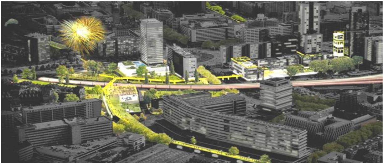
Image 4.2: The yellow Luchtsingel connects the city centre with the Luchtpark Hofbogen.
