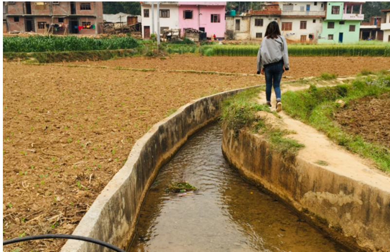
Photograph 3. Canal lined with cement. Jethi Kulo, Argali, Palpa
