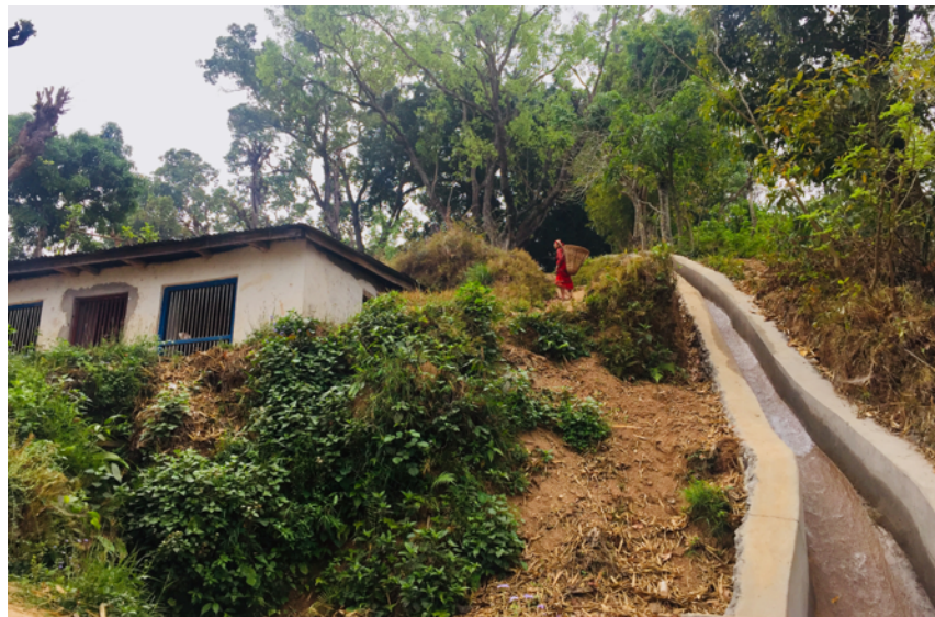
Photograph 6. View of Thulo kulo canal lined with cement. The building to the left is the community water mill
