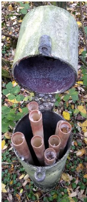
Figure 10, Monitoring well B42F0077 comprising eight tubes with varying filter depths
