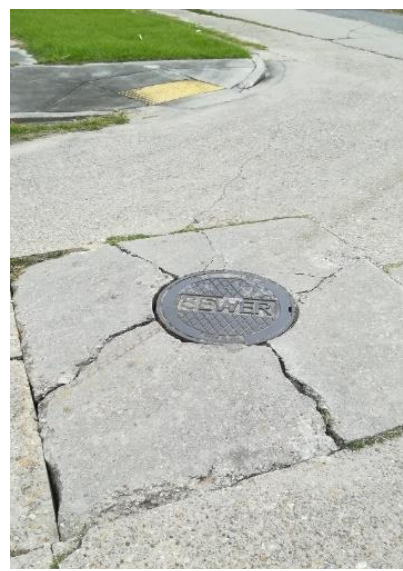
Figure 6.2.3: around paved structures the road has subsided (St. Anthony, London Avenue outfall Canal)
