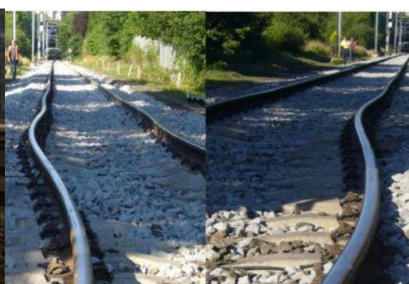
Figure 5.1.7: If outside temperature rises above 25 °C, the railtrack could be heat up to 70 °C causing rail buckling. Source: (Prorail, 2015).
