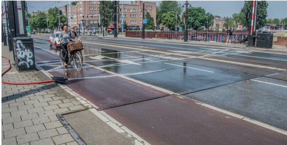
Figure 5.1.4: Bridges are kept wet to prevent steel expansion. Source: (Watersportverbond, 2018)
