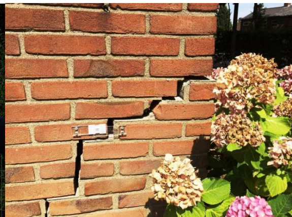
Figure 5.2.3: Tearing in walls as a result of land subsidence in Zevenaar. Source: (Opten, 2018)
