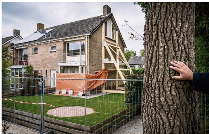
Figure 5.2.2: As a result of land subsidence, two houses have been stabilized to prevent collapsing. Source: (Schreuder, 2018)
