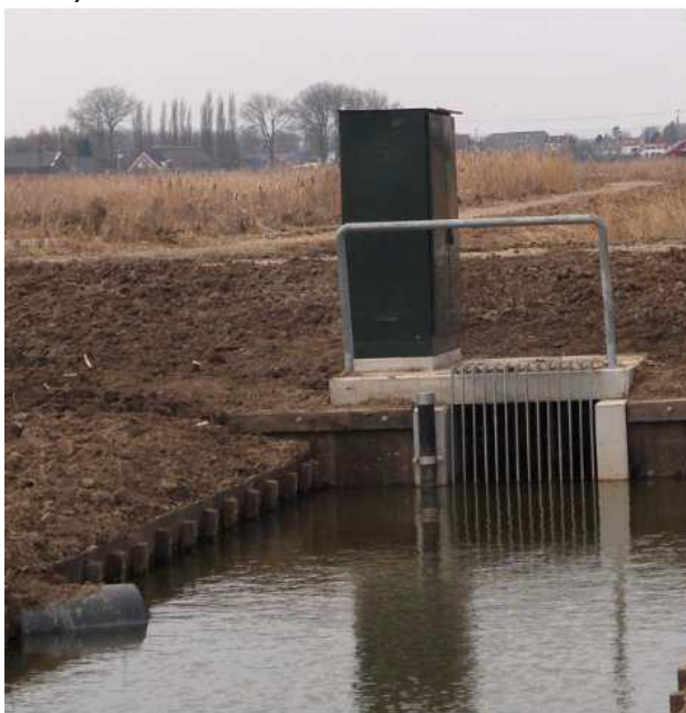
Figure 9 pumping station (department RA, 2019)
