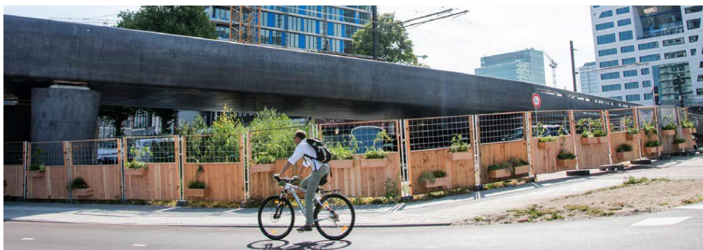
Figure 5: Green Construction Fences (YP2019)
