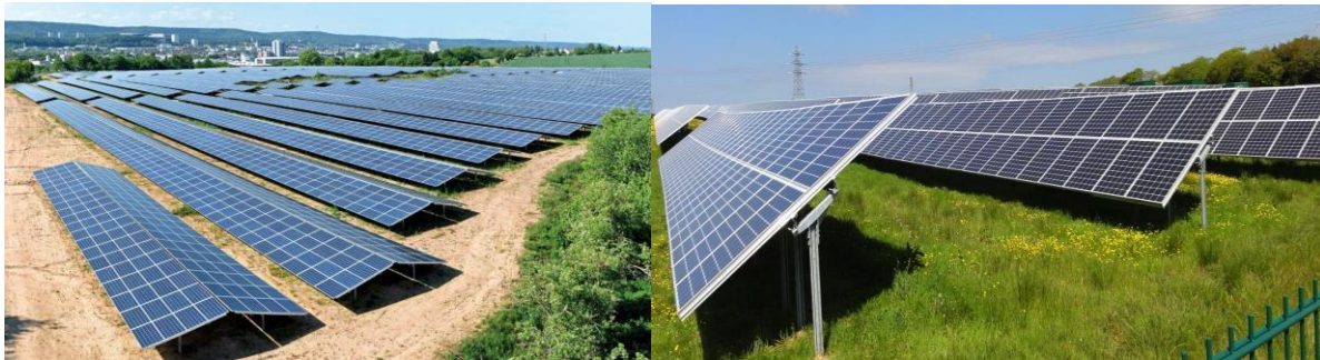
Figure 1. Examples of east-west oriented and south oriented large ground mounted solar PV systems.
