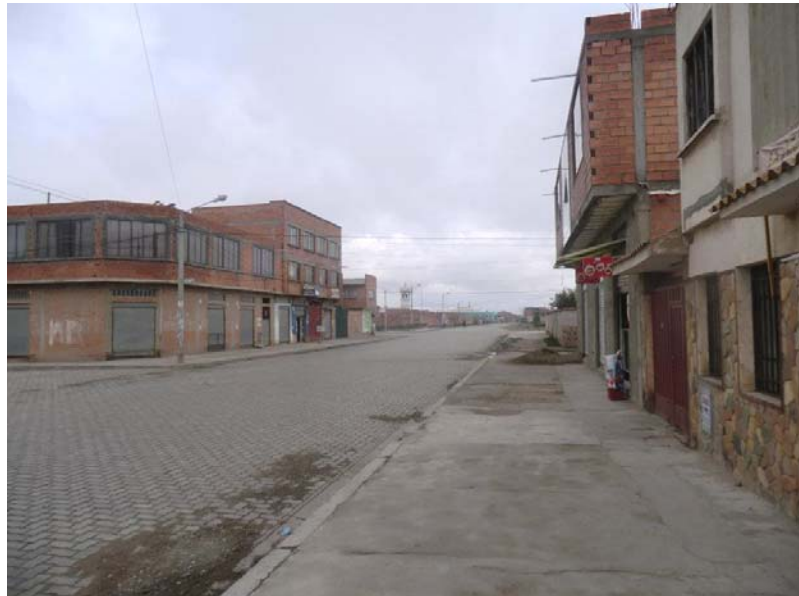
Figure 2.5. A typical street in Villa Adela, El Alto.
