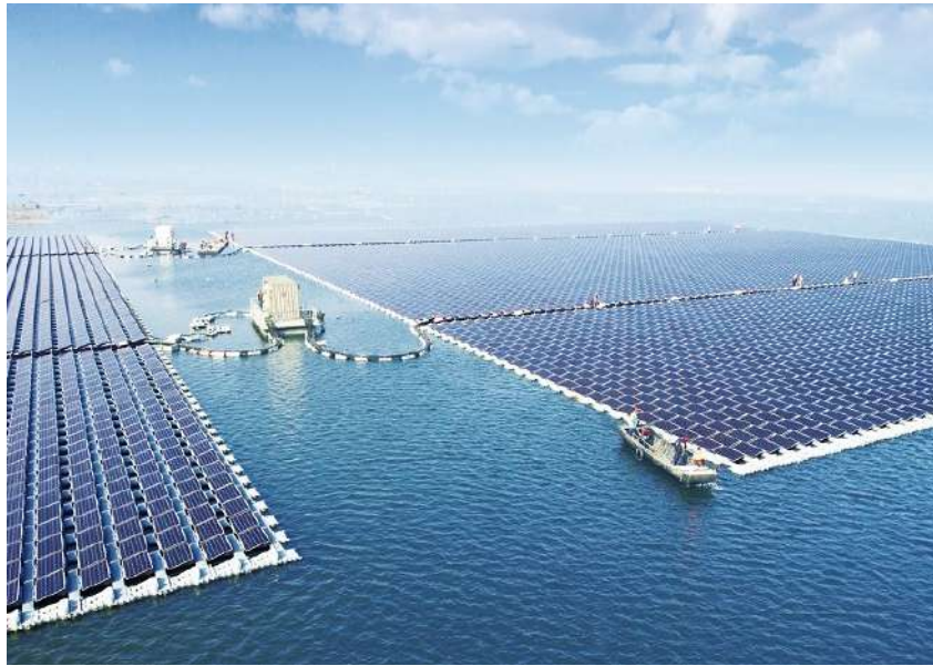
Figure 1: Image of an inshore floating solar park at Huainan, China. https://interestingengineering.com/china-powered-worlds-largest-floating-solar-power-plant
