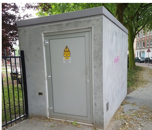
Fig. 1.1: A Ring Main Unit of Stedin in a street somewhere in Rotterdam.
