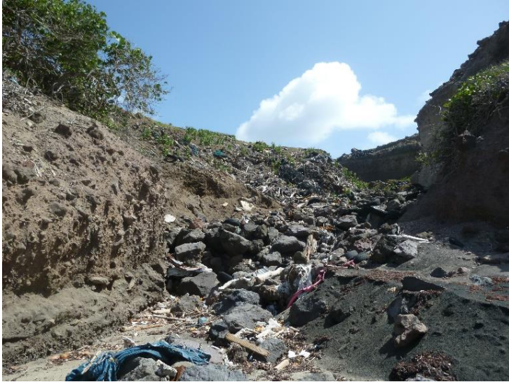
Figure 5.2: Gully erosion of coastal cliff, located at 17°30.011' N 062°58.310' W.
