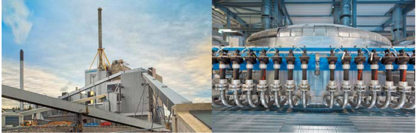
Figure 7. The Lahti Energy Kymijärvi II waste gasification plant (left) and gas cleaning filter (right).
