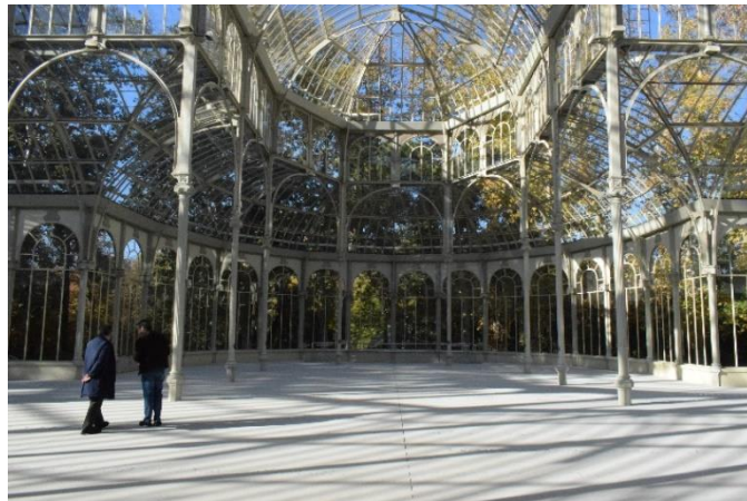
Figure 10. The view inside the Crystal Palace at El Retiro Park, Madrid, Spain. (Photo by D. Wilson)
