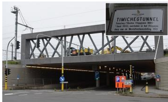
Figure 27. Timicheg Tunnel, Ghent, Belgium. (Photo by D. Wilson)
