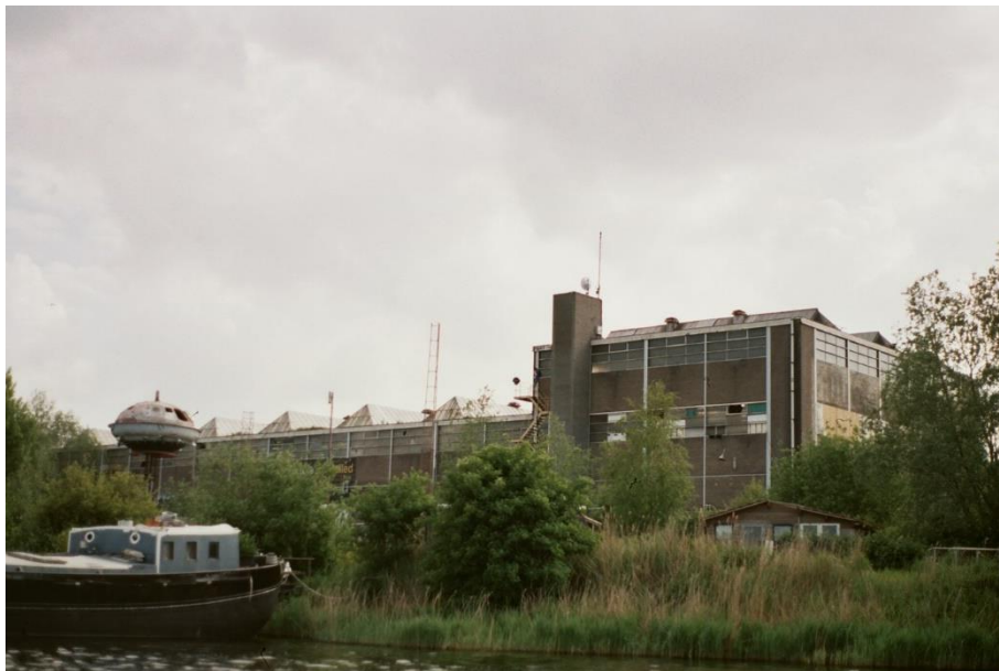
Figure 17: ADM as seen from the water. Shot on 10-5-2018
