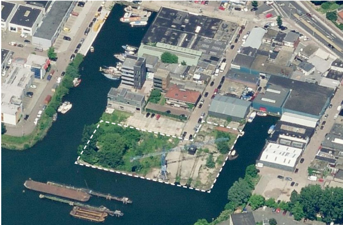
Figure 2: De Ceuvel is build on a former ship wharf
