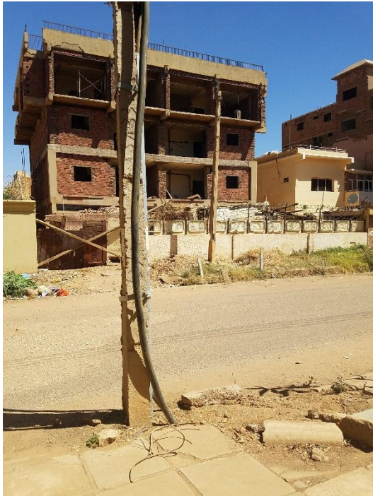
Figure 15 Stalled construction site in al-Amarat, that housed squatters turned guardians.
