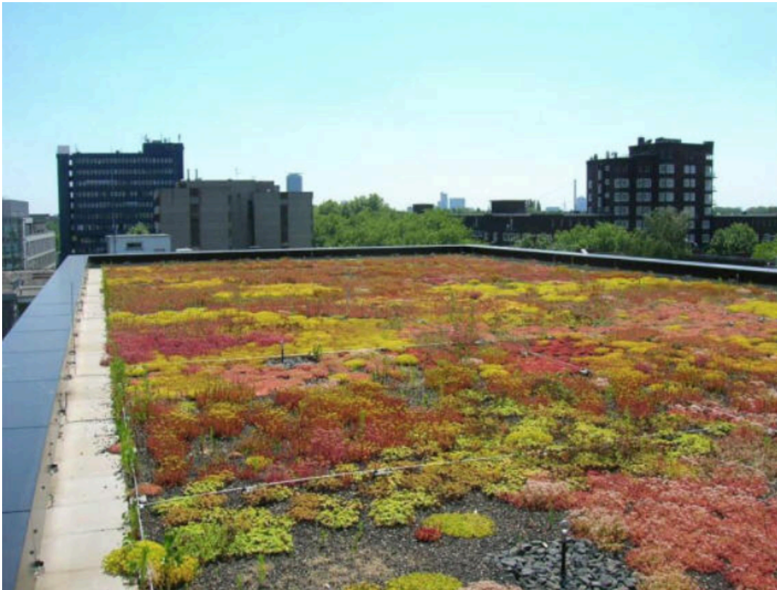
Figure 3. An extensive green roof covering 7,000 square meters in Düsseldorf, Germany (source: http://www.greenroofs.com/content/guest_features006.htm )
