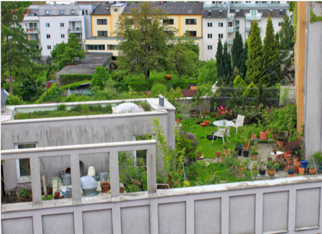
Figure 2. An intensive green roof garden in Linz, Austria (source: https://livingroofs.org/intensive-green-roofs/ )
