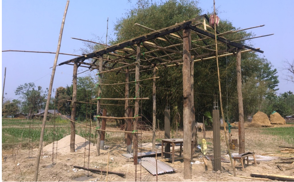
The early construction of a home in Jhapa using locally sourced timber. Author's own.
