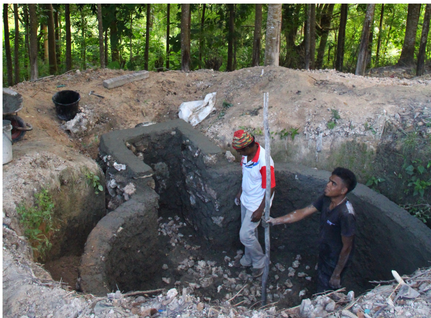
The construction partner organisation building a domestic bio-digester.
