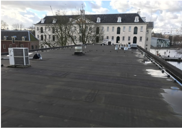
Figure A1 Bitumen roof, before construction of the green roof.
