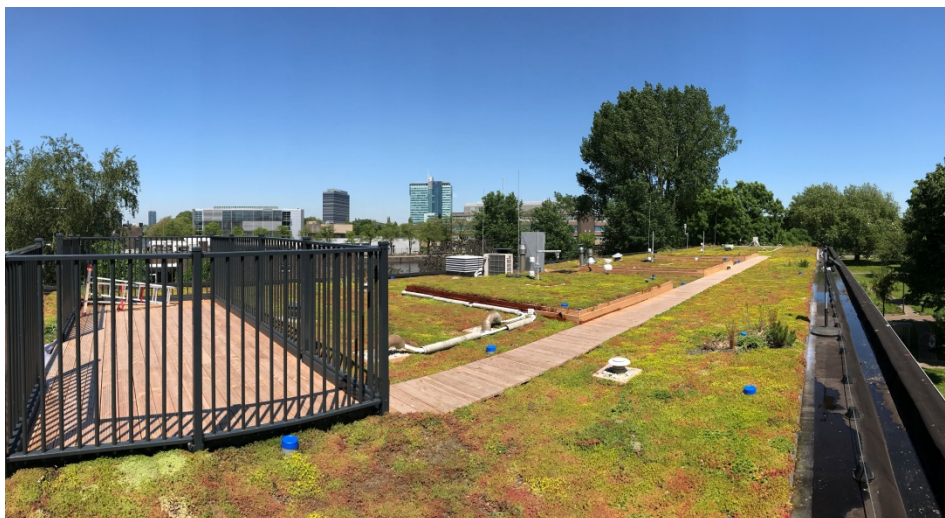
Figure A5 After construction of the green roof
