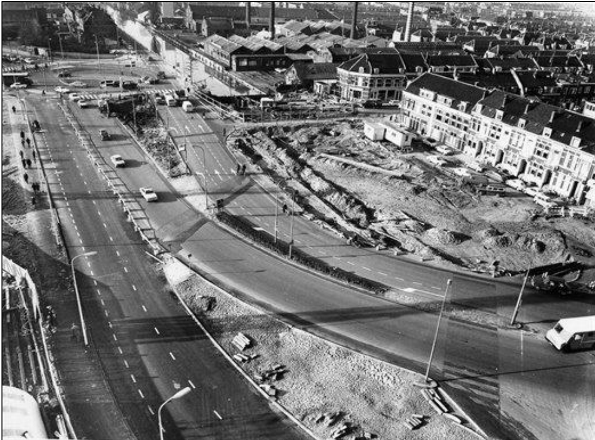
Figure 4-2: Construction of Westplein in 1969
