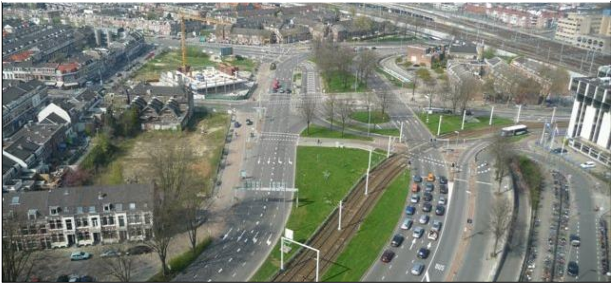
Figure 4-3: Westplein from above 2010 (Source: CU2030.nl)
