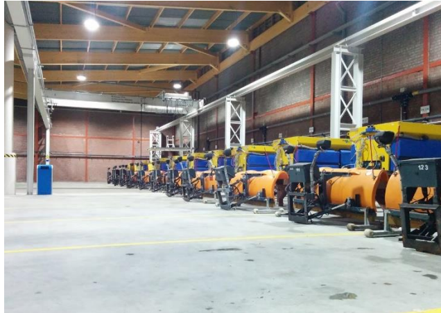
Figure 4.6 Depot Giessenweg [author's own picture]
