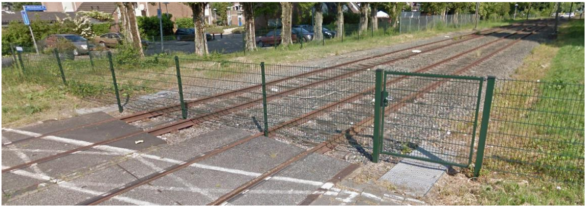
Figure 13. Closed rail crossing
