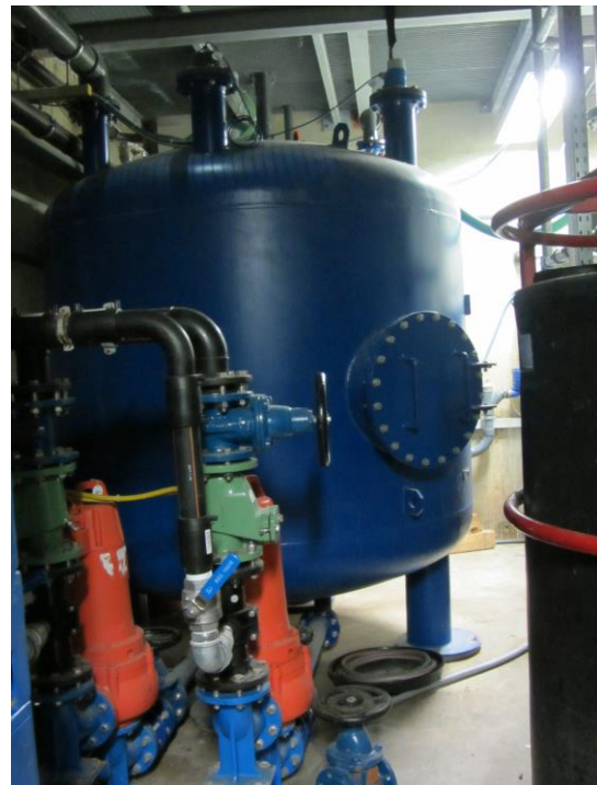
Figure 4.9 The subterranean collection chamber
