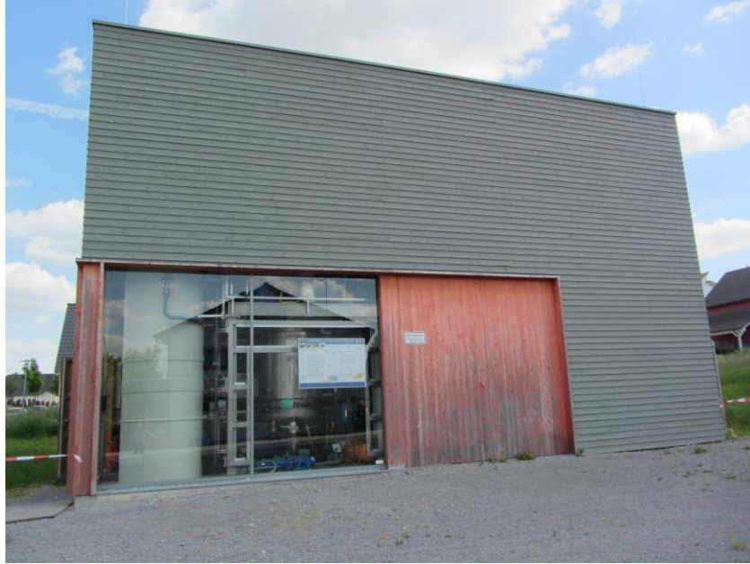
Figure 4.10 DEUS 21 Waterhouse , containing the wastewater treatment modules
