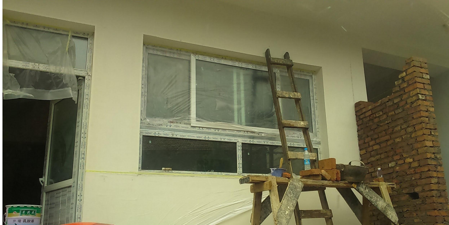
Figure 11. Energy efficiency improvement in door and windows, Caocangcun. July 15, 2017.
