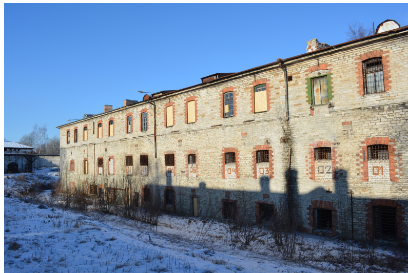
Image 3: Photo of the altered façade. 100
