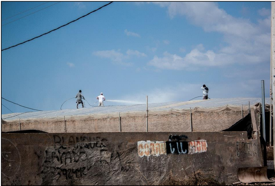
Picture 6: Three greenhouse workers spraying white paint on top of a greenhouse.
