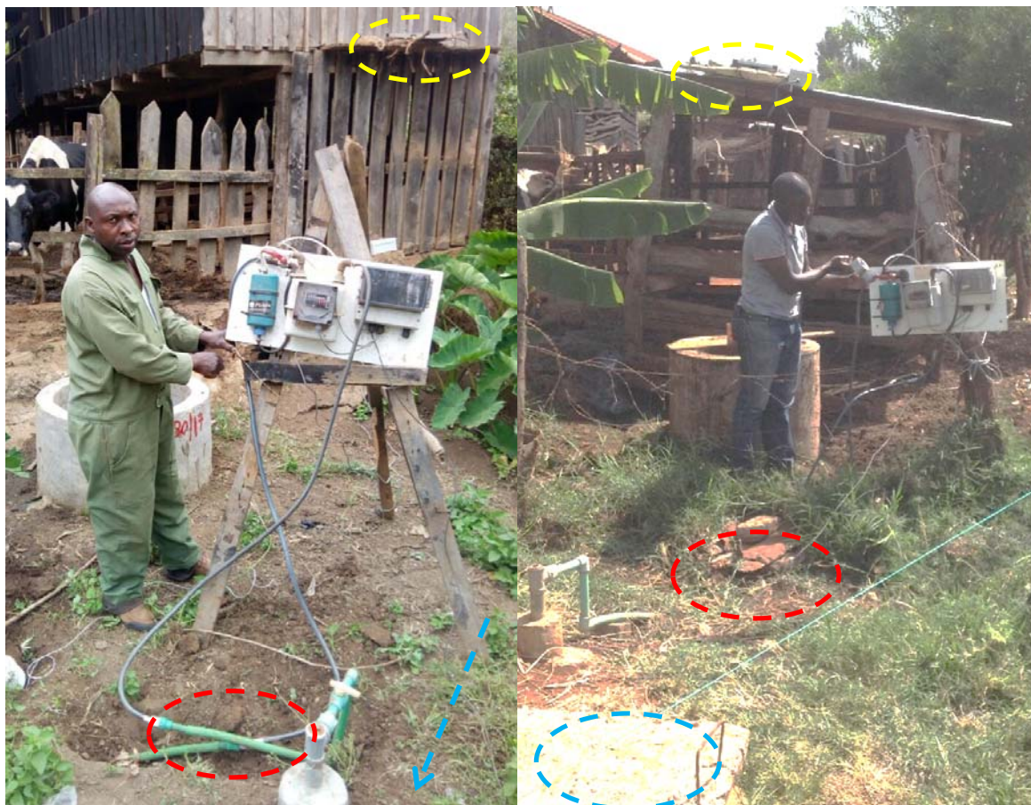
Figure A 8: examples of the positioning of the data logger for biodigester 6 (left) and 3 (right). The position of the solar panel is marked by a yellow circle. The red circle shows the spot where the biodigester piping is interfered for connecting the data logger. The blue circle represents the location of the expansion chamber, where the temperature sensor is inserted. Picture from own archive.
