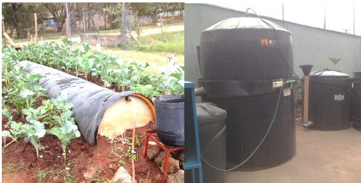
Figure 5: picture of the Rehau bag digester type (left) and two versions of the Blueflame floating dome type (right). Pictures from personal archive.
