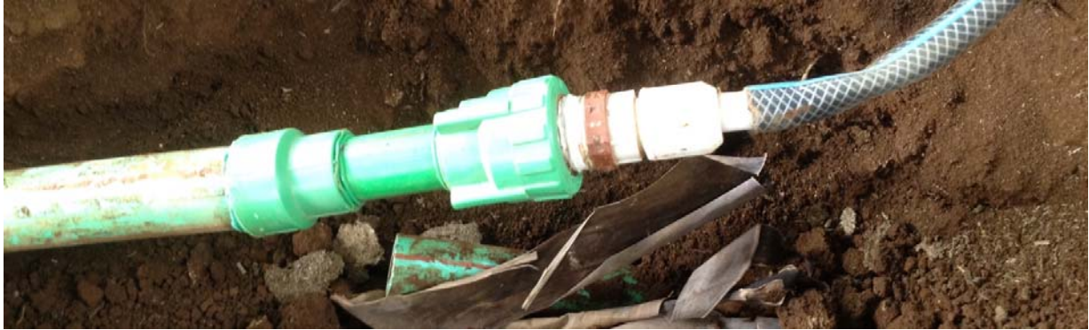
Figure A 9: example of a welded connection of the biodigester piping (left) to the hose that connects with the data logger (right). Picture from own archive.
