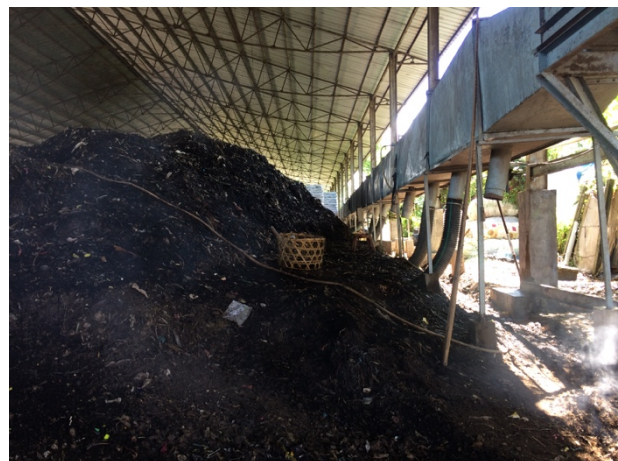
Figure 20: Aerobic composting at Temesi
