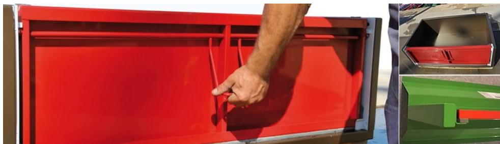
Figure 3.19. Installing of anti-flood barriers
