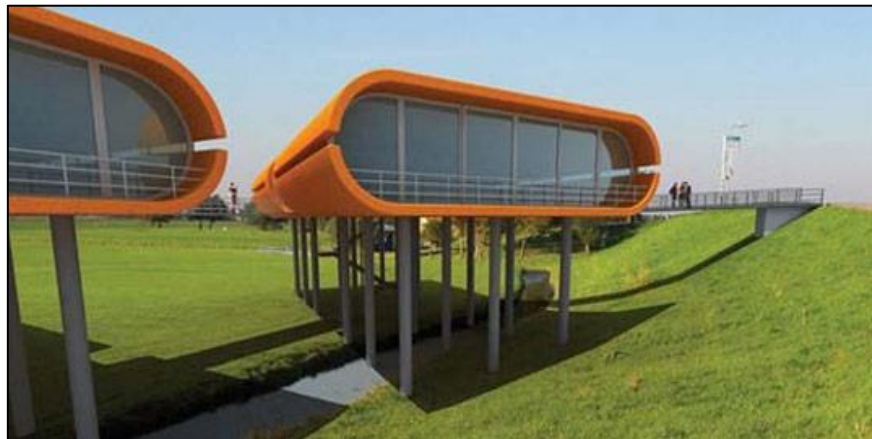
Figure 3.19. Flood prove housing
