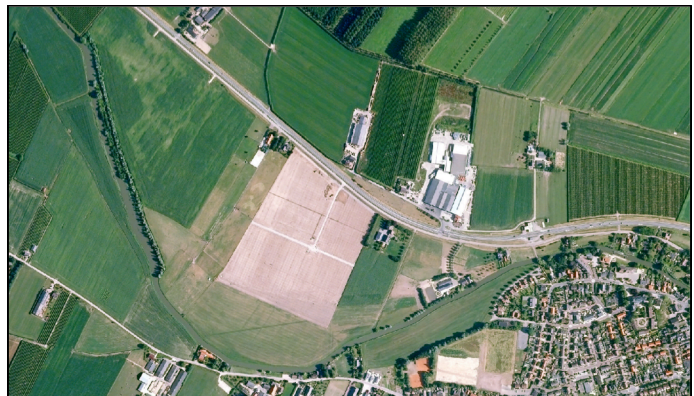
Figure E.1. Project location in 2009
