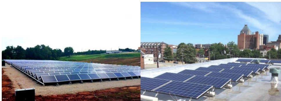
Figure 2.1: V-shaped (left) and South-facing (right) solar panels.
