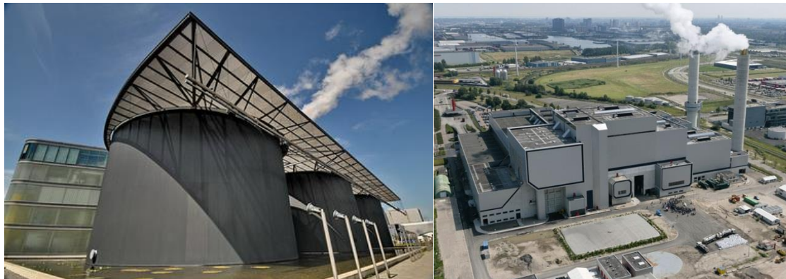
Figure 1.4: Left, Amsterdam West's digestion tanks ( www.wabag.com ); right, AEB's incinerator ( www.aebamsterdam.com ).
