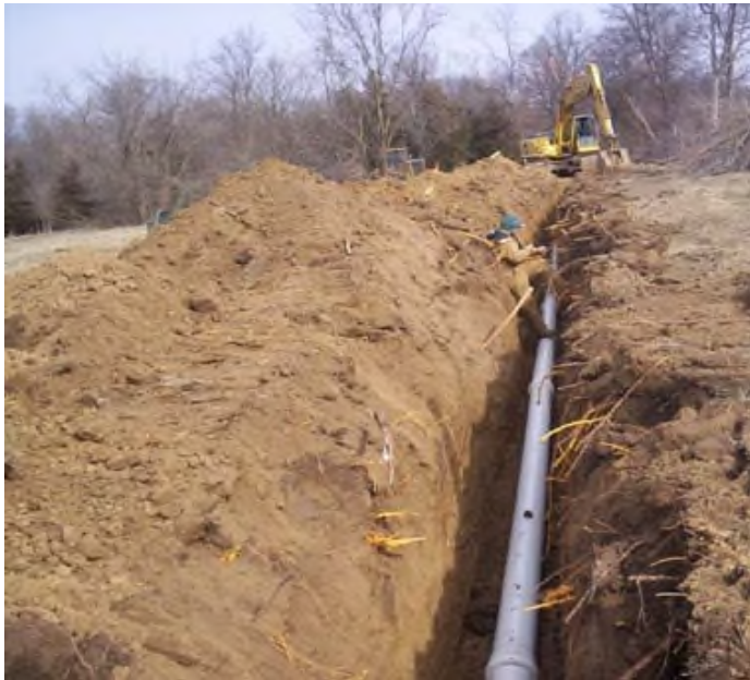
Figure 2-1: Open-cut for installation, replacement or rehabilitation
